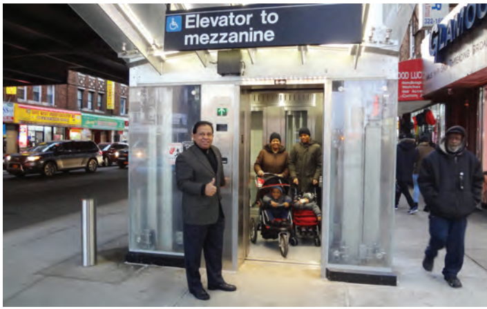
A determined push by community leaders brings elevator to A Train Station Lefferts-Ozone Park. Community advocate Albert Baldeo opens the door for the babies and parents to access the A train.
