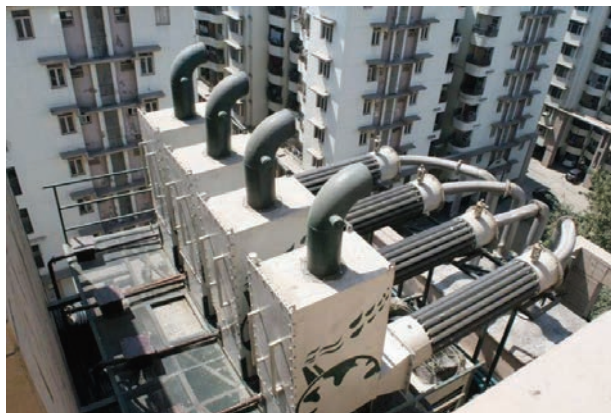
A device created by company Chakr Innovation to remove soot from diesel generator exhaust, to clean the air and to allow ink to be created from soot.
