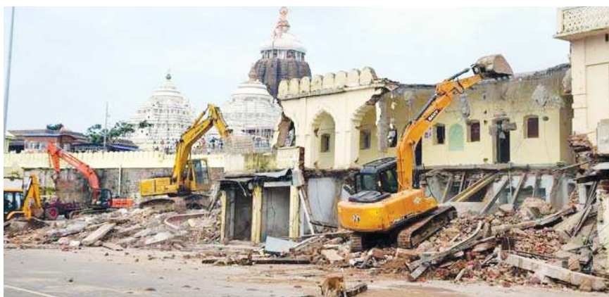
Historic mutts around Jagannath Temple being demolished.
