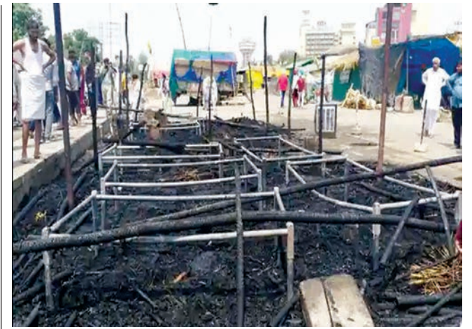
The tents damaged in fire at the Singhu border on April 15.
