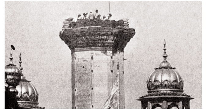
The historic Ramgarhia Bunga damaged in the Operation Bluestar - Photo / Courtesy Central Sikh Museum.com
