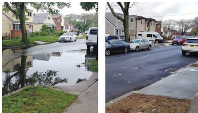
Prior to construction, stormwater would collect on 160th Street between 132nd Avenue and 134th Avenue for days (left). Since new streets and storm sewers were installed, the same location has remained clear (right).
