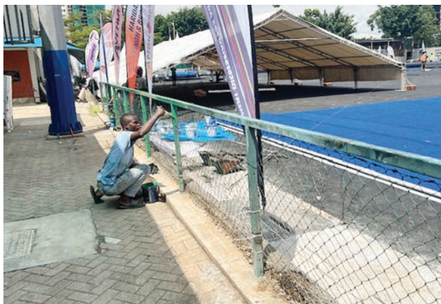
Final touches to the Hockey Stadium
