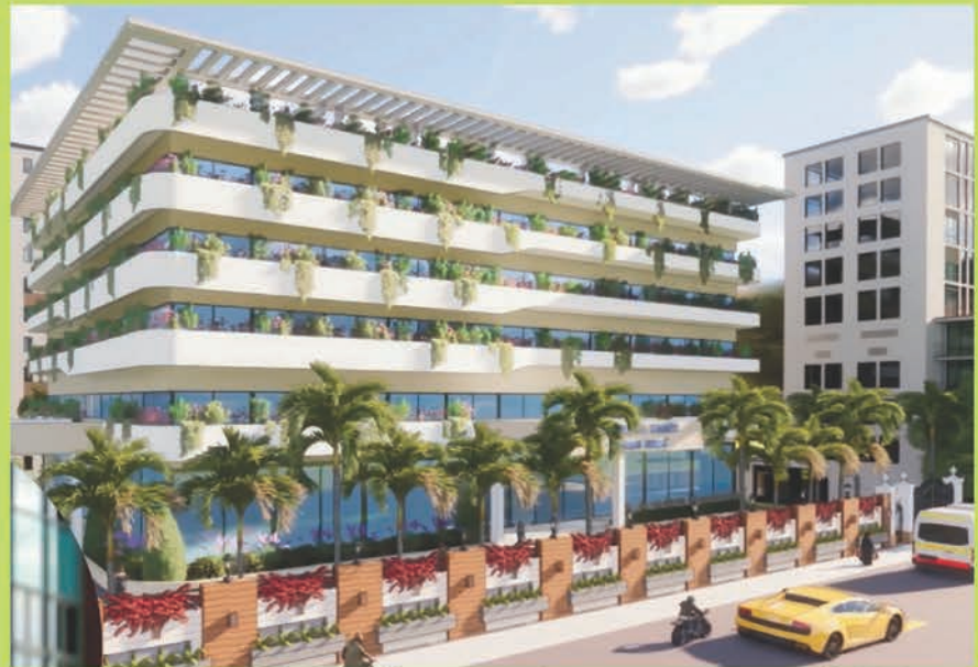
New Goutami Institute to be constructed 2024
