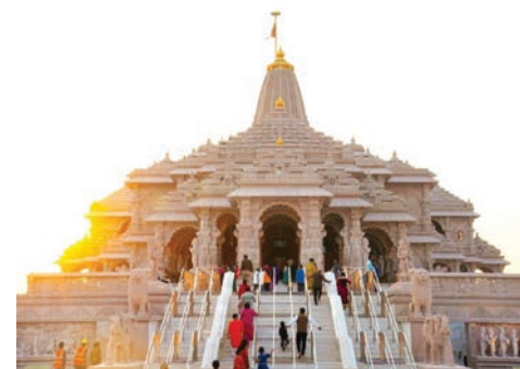
A view of Ram temple in Ayodhya. Photo: X/@ShriRamTeerth
