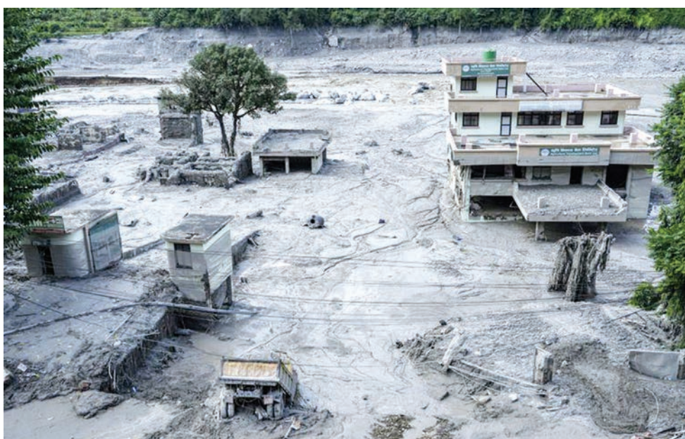
Damaged houses stand precariously near the swollen, debris-choked banks of the Trishuli River after flash floods in Nepal's Nuwakot district on Wednesday, Aug. 26, 2026. -Photo/Niranjana Shrestha
